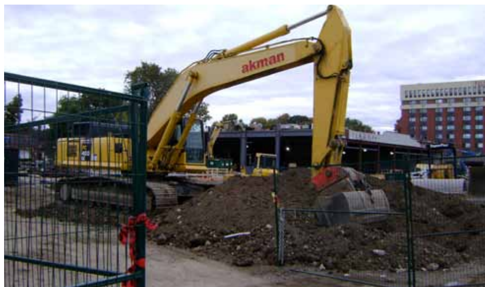
The construction site on a quiet day.
